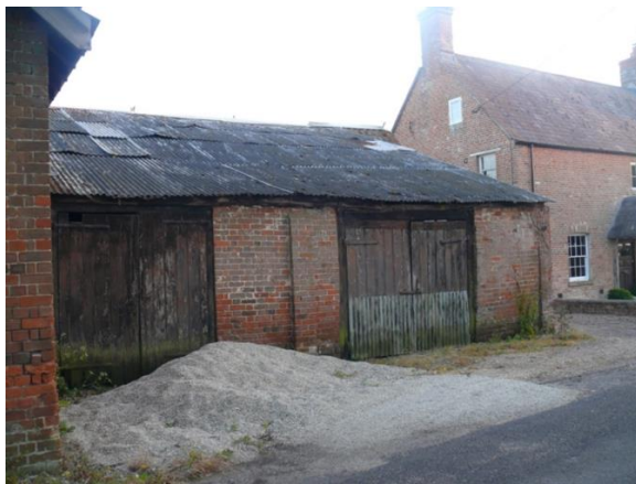
Northern elevation of building 2
