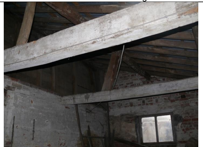
Western interior of building 2
