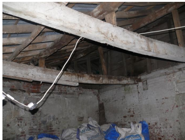
Eastern interior of building 2
