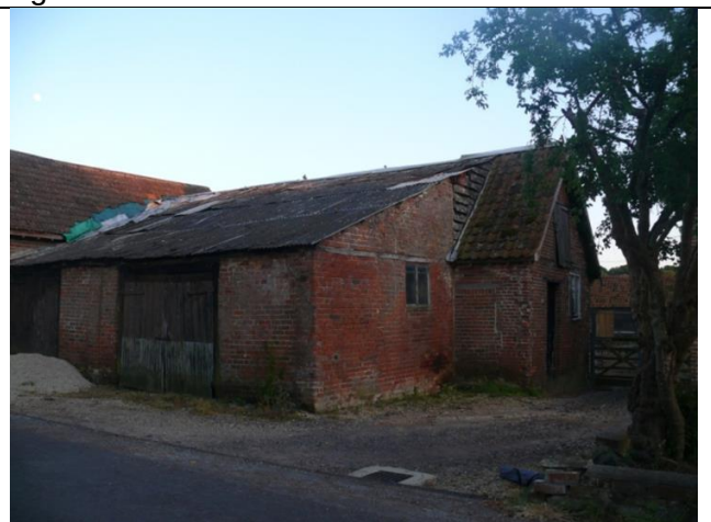
Western elevation of building 2 showing intersection with building 3
