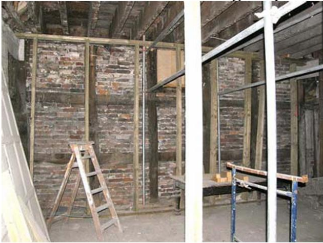
East wall (F10)
