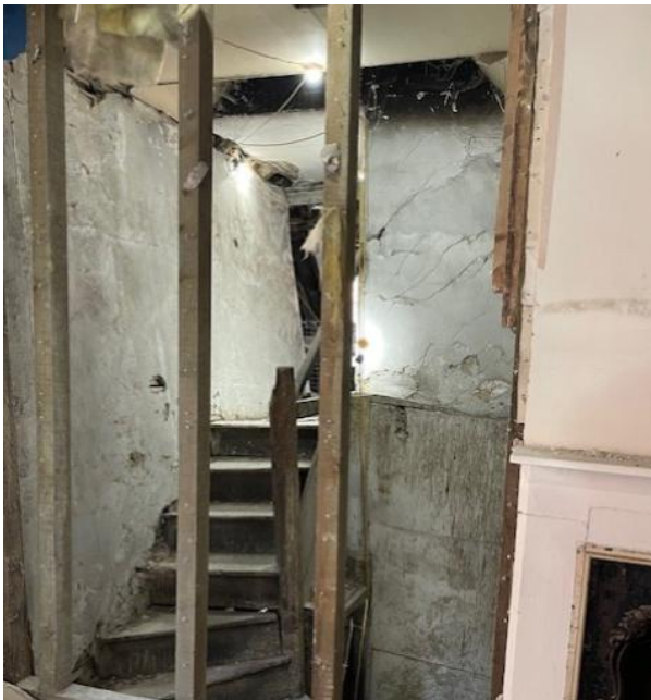
Lathe and plaster lining the hall sides
