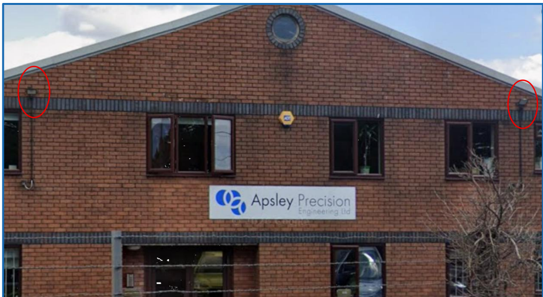
Figure 6: View of lighting at High Post Business Park
