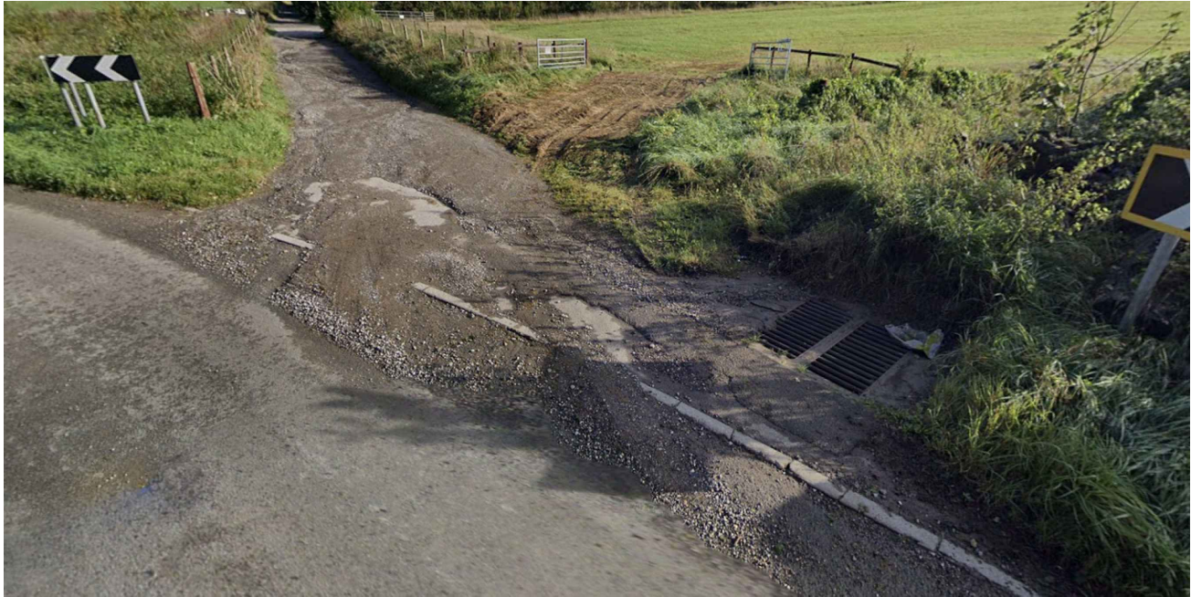
Proposed North entrance to site showing location of existing road gully and surfacing. Photo NTS
