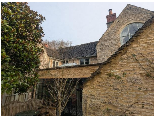
Figure 6. Southwestern and southeastern elevations of the dwelling
