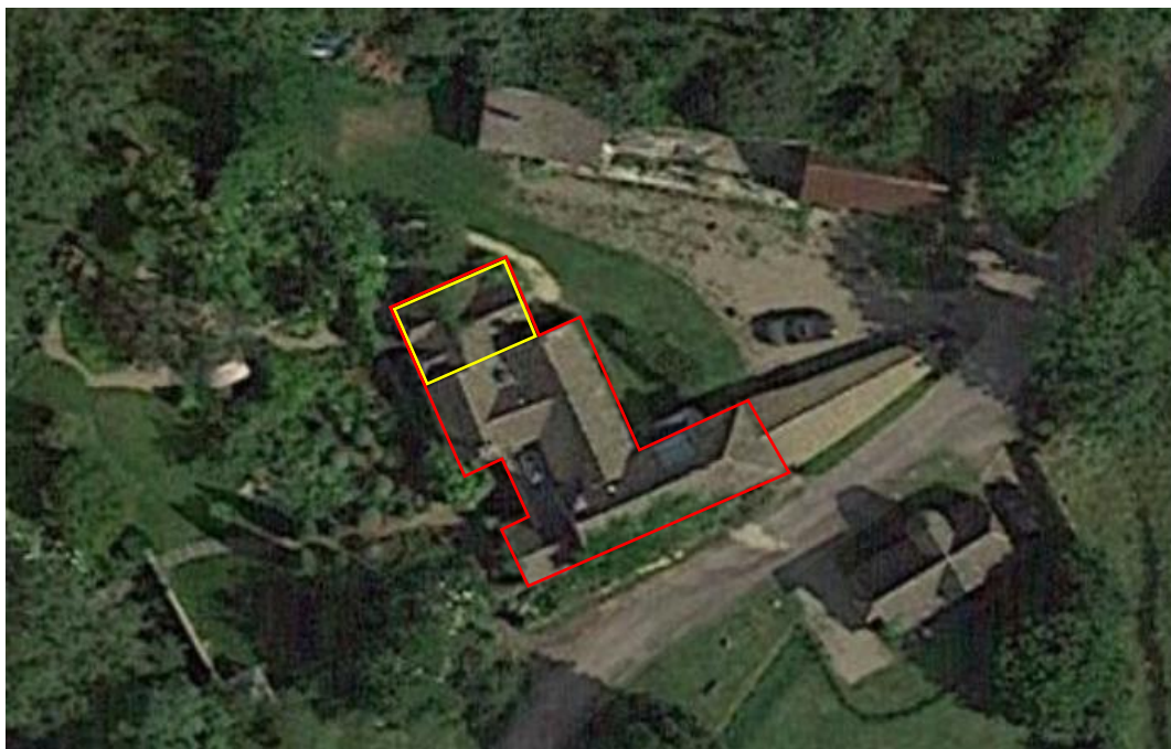
Figure 1. Goulters Mill, Nettleton (dwelling outlined in red, northwestern extension outlined in yellow)
