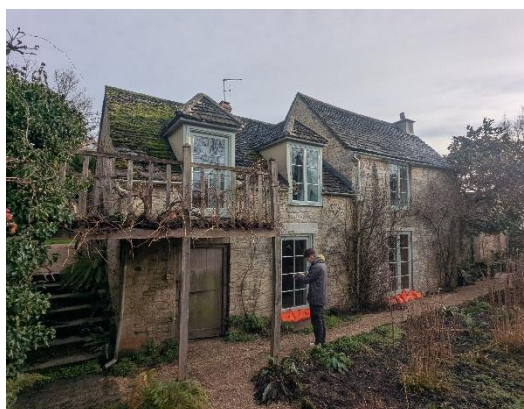
Figure 5. Southwestern and northwestern elevations of the dwelling
