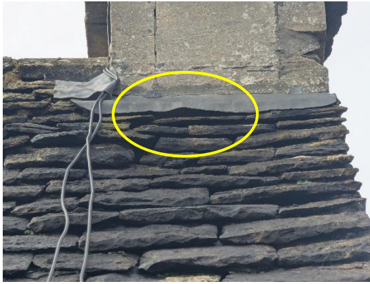
Figure 11. Potential crevice roosting position beneath the flashing on the northwestern chimney
