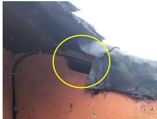
Figure 14. Potential access point at the eaves on the northeast elevation
