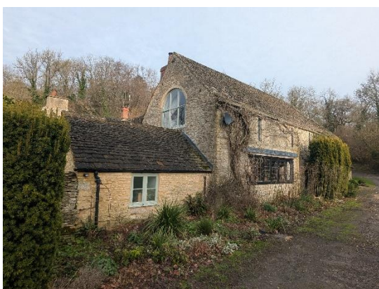
Figure 2. Southeastern and southwestern elevations of the dwelling
