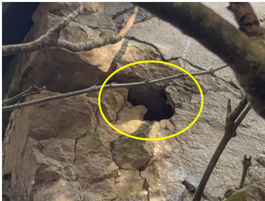
Figure 13. Potential access point on the southwestern elevation
