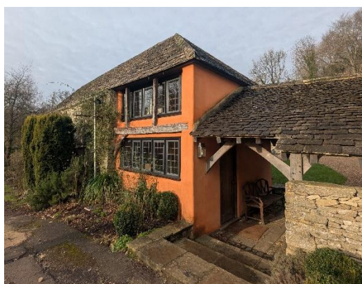
Figure 3. Southeastern and northeastern elevations of the dwelling
