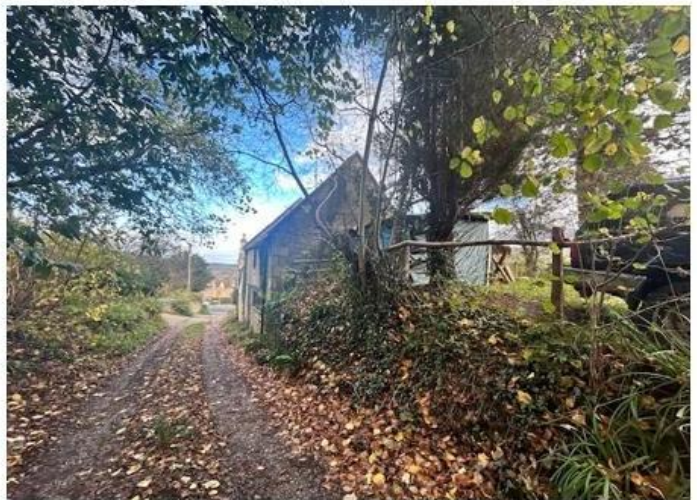
Below: South elevation and view down byway
