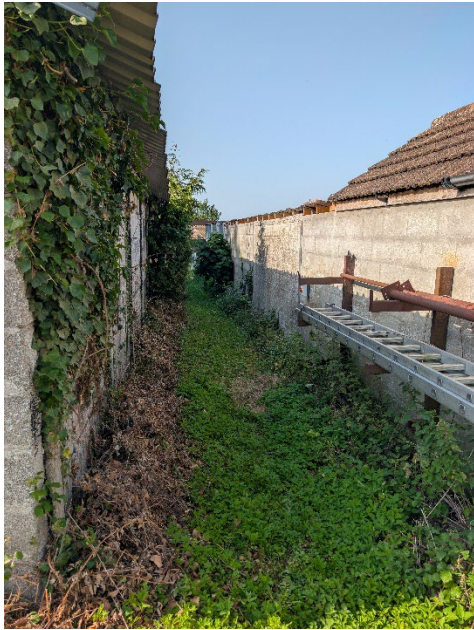
Figure 2 From the front corner of the outbuilding. AC unit to be sited behind ladder rack.
