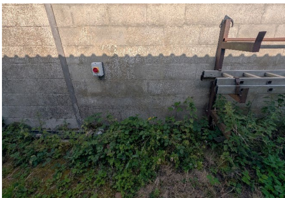
Figure 1 Location of proposed AC unit, adjacent to ladder rack.
