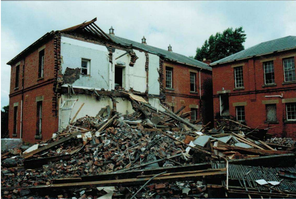
2003 view of the application building from the south-east, showing the two service wings (one in place and one demolished). The main elevation was then completely remodelled.
