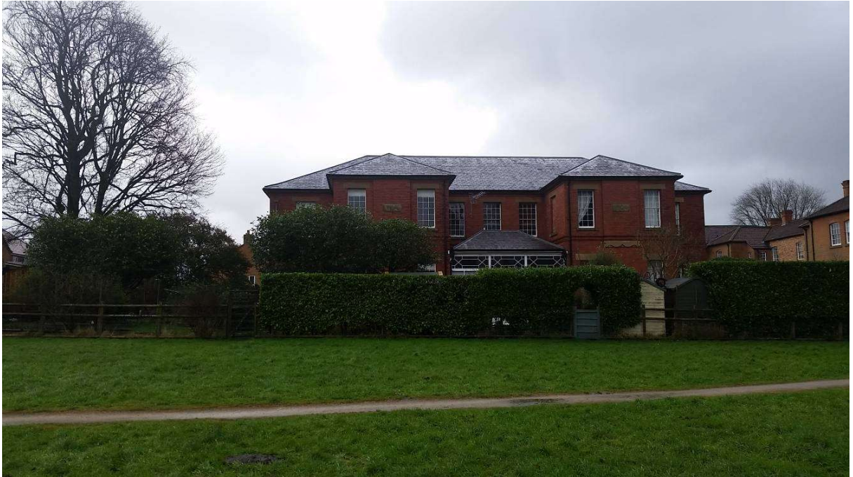
Existing view of the west elevation. The extension would be hidden from view, behind the hedge on the right of the picture.
