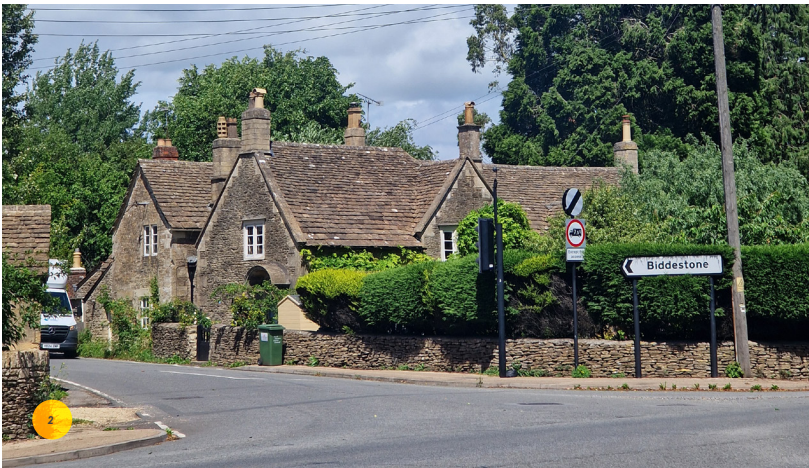
FIG 1. VIEW LOOKING TOWARDS HOUSE FROM MAIN ROAD TO SOUTH EAST ELEVATION
