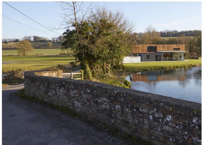
Werg - Contemporary Timber Architecture Flat roof and asymmetrical roof
