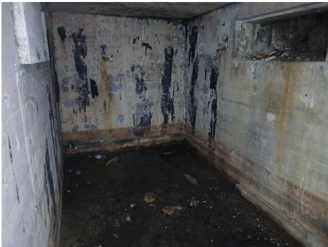
Photo 13: Second chamber B2.
