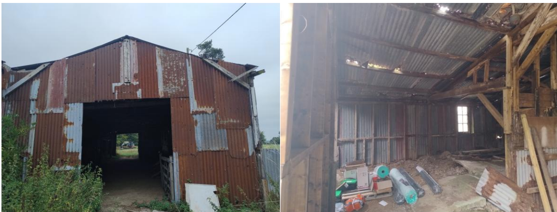
Figure 5 and 6: Images of the barn
