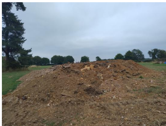
Figure 2: Spoil heap present due to current works
