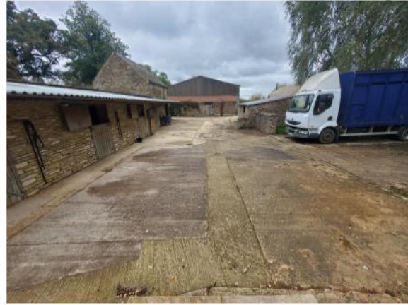
Photo 8: A view of the hardstanding yard located to the immediate south of the stables.
