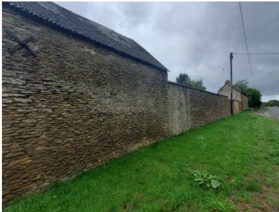
Photo 1: The northern roadside boundary wall.
