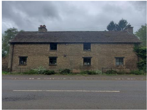
Photo 2: The north facing elevation of the residential dwelling.
