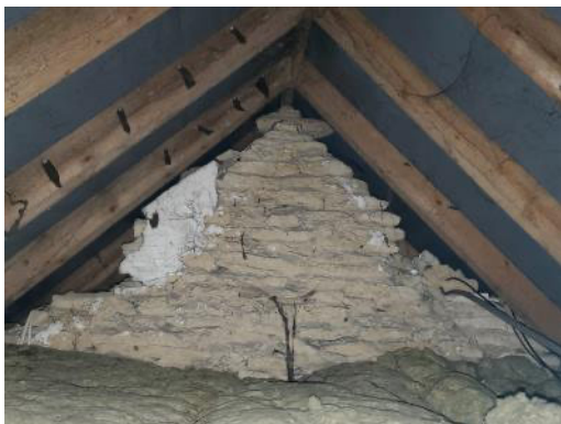
Photo 5: An internal view of one of the three loft voids.
