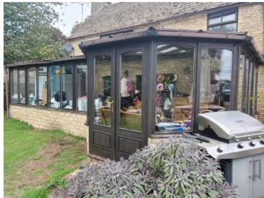
Photo 4: The conservatory which adjoins the south facing elevation of the dwelling.
