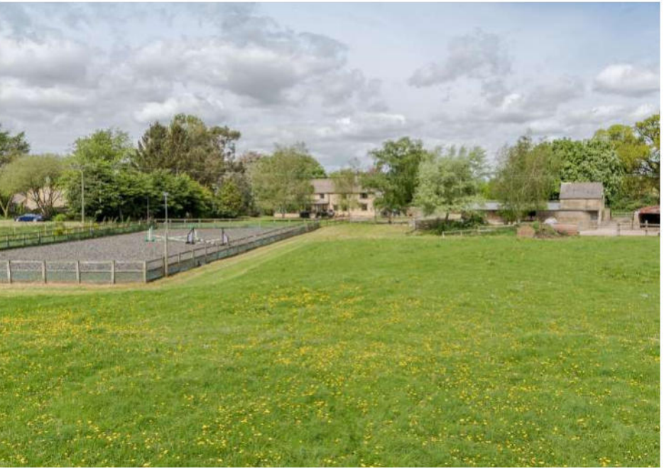
View of the existing cottage from the fields, showing menage and outbuildings etc
