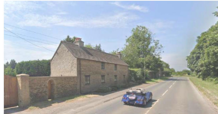
View of the existing cottage condition and proximity to the road
