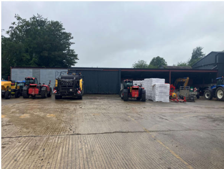
View of the existing implement shed from the east
