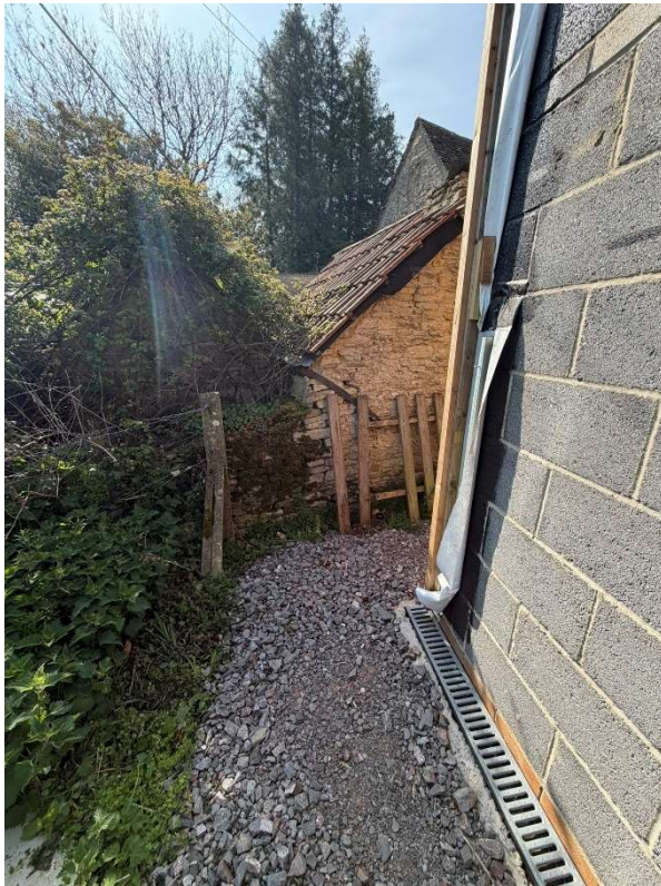
Image 6: View of rear of building with neighbouring property
