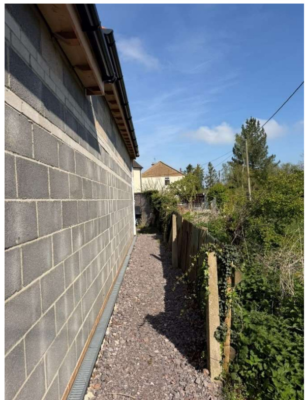
Image 7: View along rear wall and site boundary
