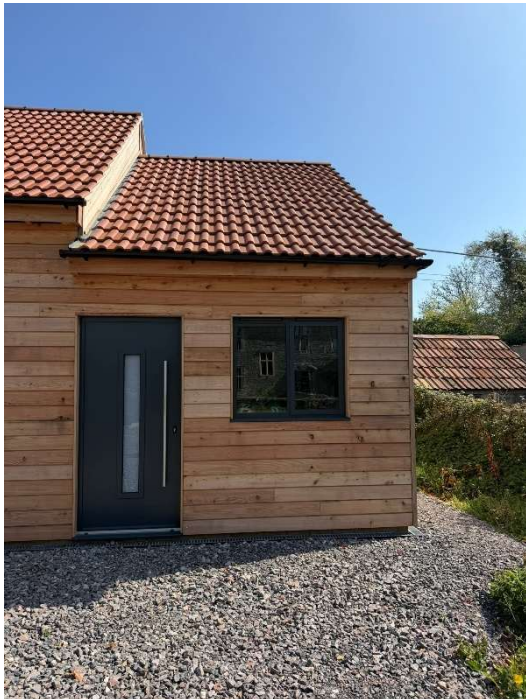
Image 3: Side of garage building in situ
