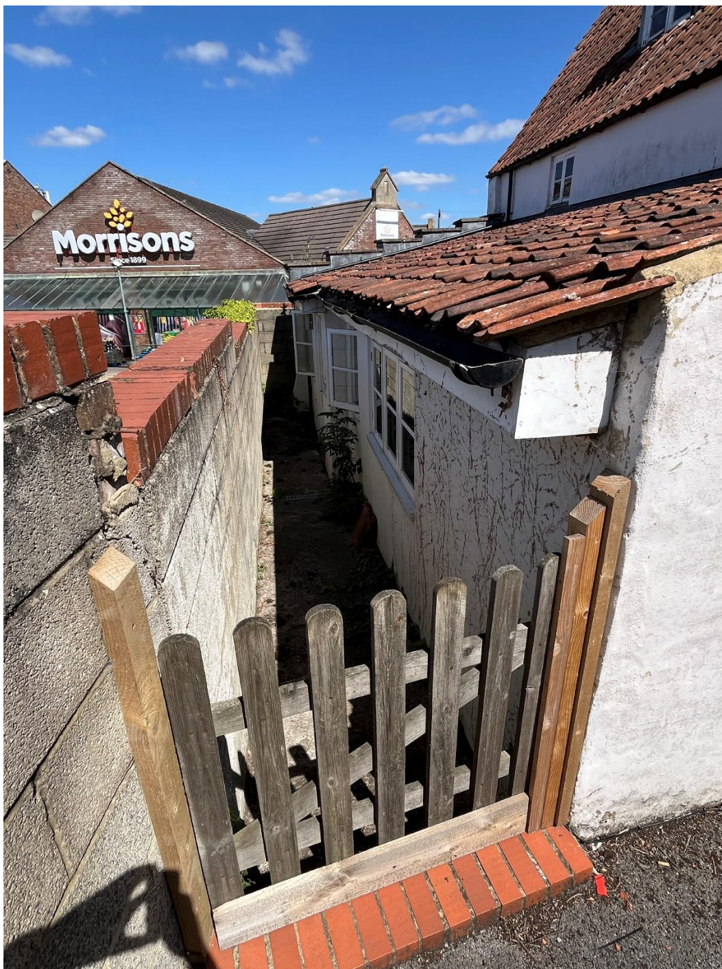
View of the eaves of the existing lean-to roof, viewed from the south. Existing pantiles are to be replaced with natural slate (with a hidden waterproof backing system). All other details to be retained as existing.
