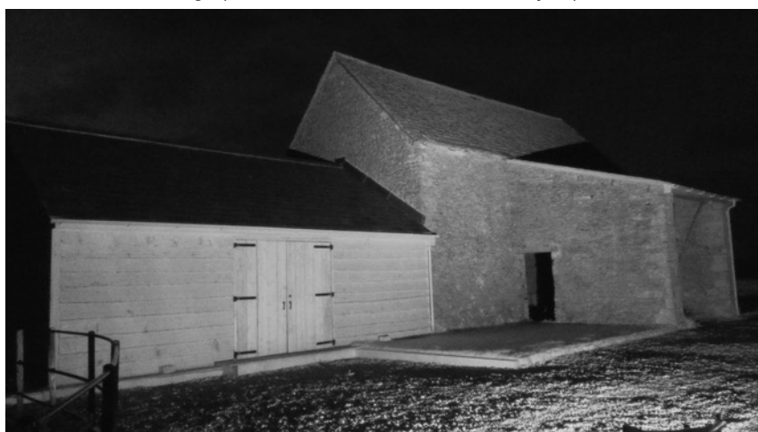
Photograph 3: View of the barn from surveyor position 2.
