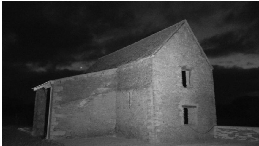
Photograph 1: View of the barn from surveyor position 3.
