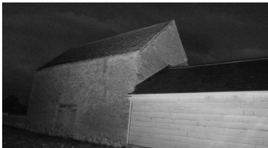
Photograph 2: View of the barn from surveyor position 1.
