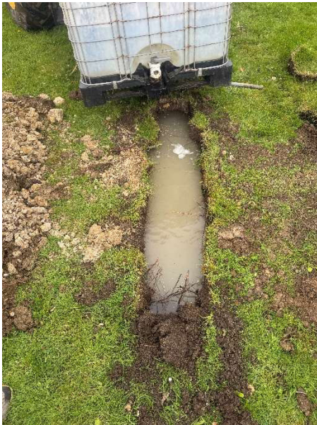
Picture 1 – Start of test
