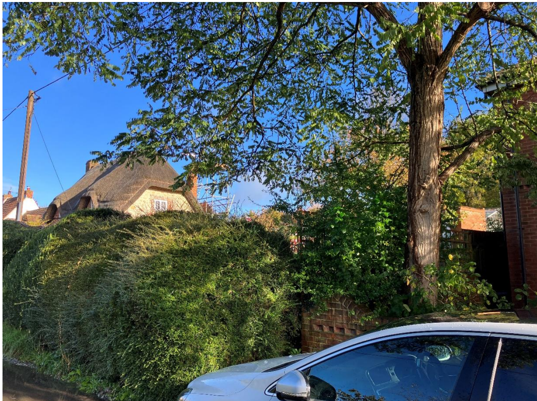
Fig.01 Looking towards Box Cottage from Whistley Road
