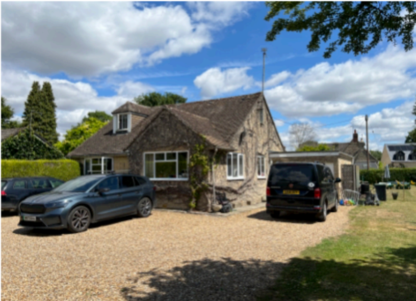
View as above, showing existing dormer
