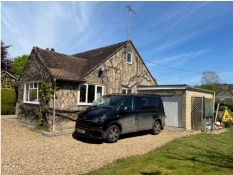
View from the south west looking towards the garage
