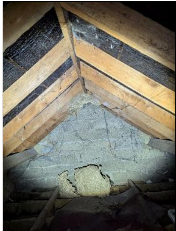
Image 2: Front void of residential building
