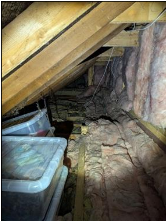
Image 1: Front void of residential building
