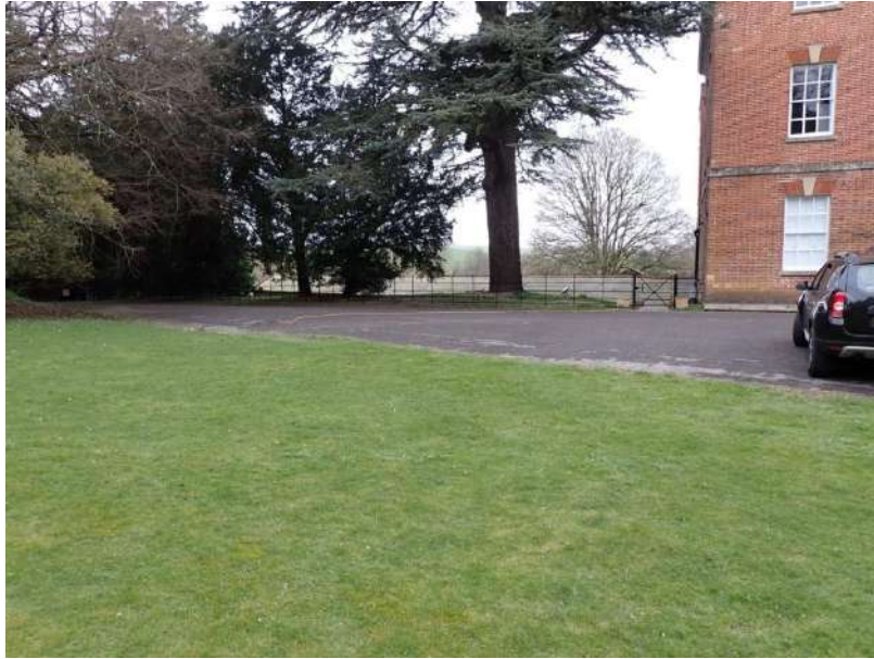
Plate 3: View of the assessment site, from the south
