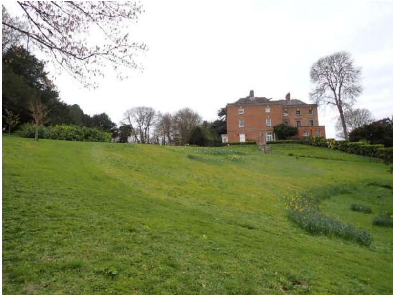
Plate 68: View of the assessment site, from the east
