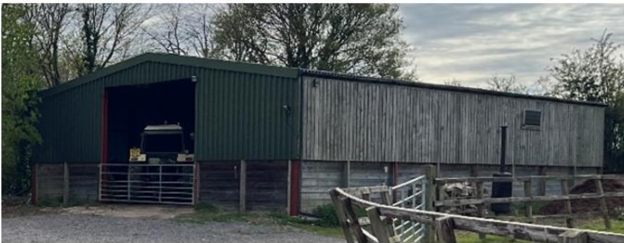
Case officer's site photos of the existing barn
