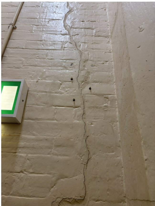
P45 – Crack gauges under monitoring.
