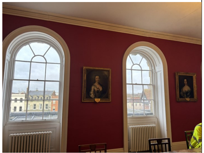
P14 – Georgian arched sash windows in Grand Jury Room.
