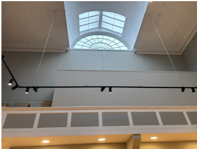
P21 – Principle crack as seen from ground floor.
