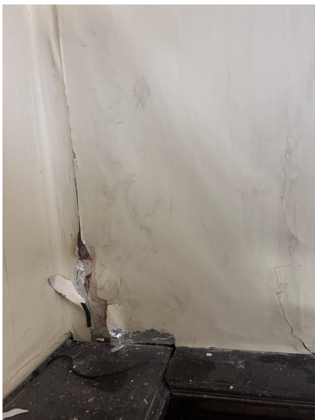
P41 – Paper physically feels fine and no deterioration noted suggesting that the water ingress has been repaired.
