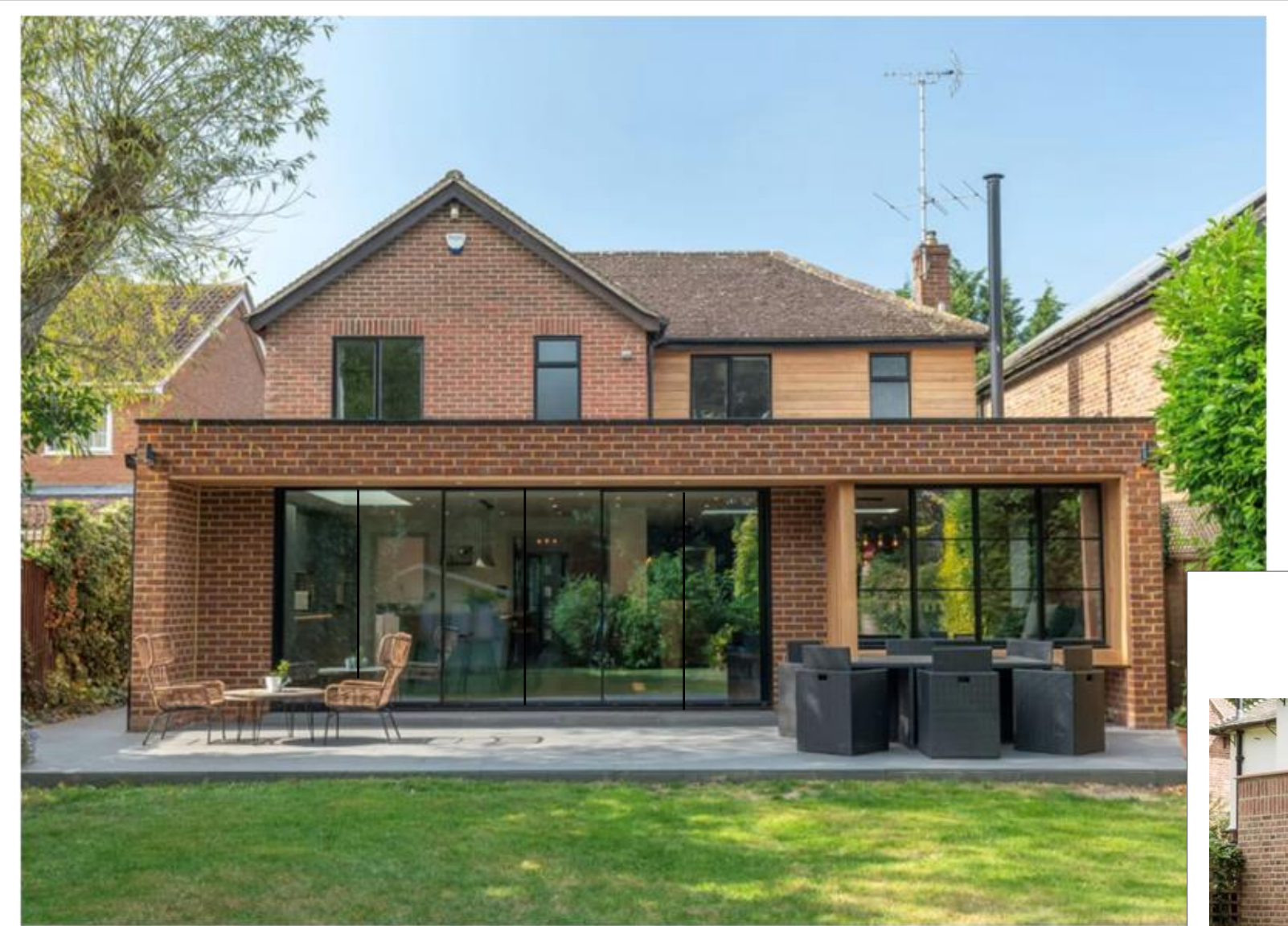
Flat roof ground-floor extension with recessed glass 'wall' of doors to garden
