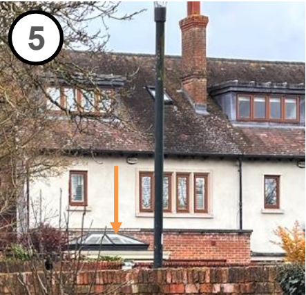
5. Glass roof lanterns, Cromwell Court (seen from Priory Gardens)
