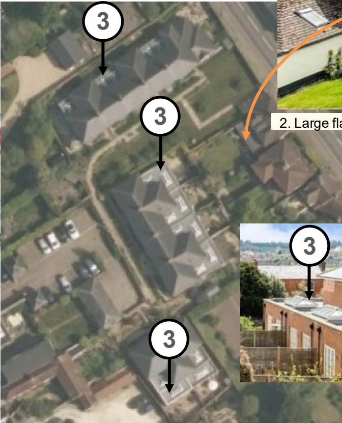
3. Multiple flat roofs with glass lanterns at Clarendon Court
