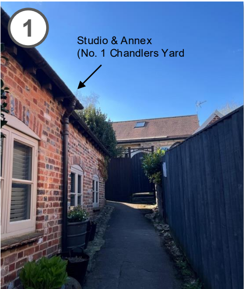
1. Entrance to south-eastern side of application site (as seen walking up Chandlers Yard from the High Street)
