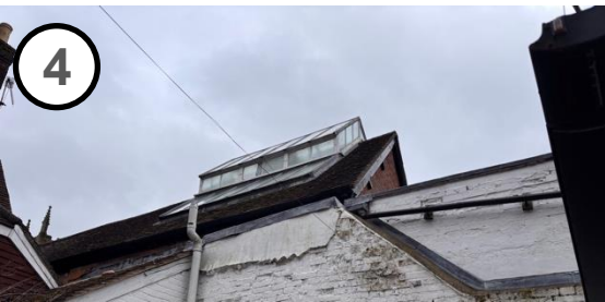
4. Glass roof lantern #5 Kingsbury Street
