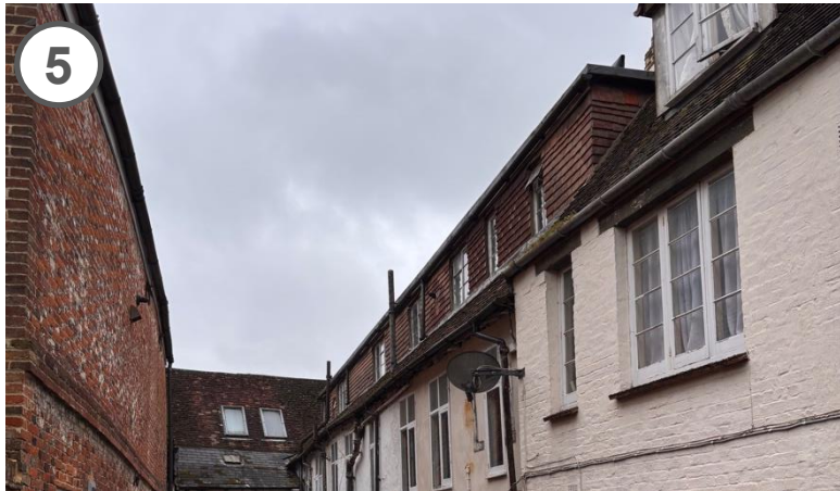
Full-width box dormer on rear extension #139 High Street (Grade II listed), easily visible from Ironmonger Lane (PRoW MARL12) 2
