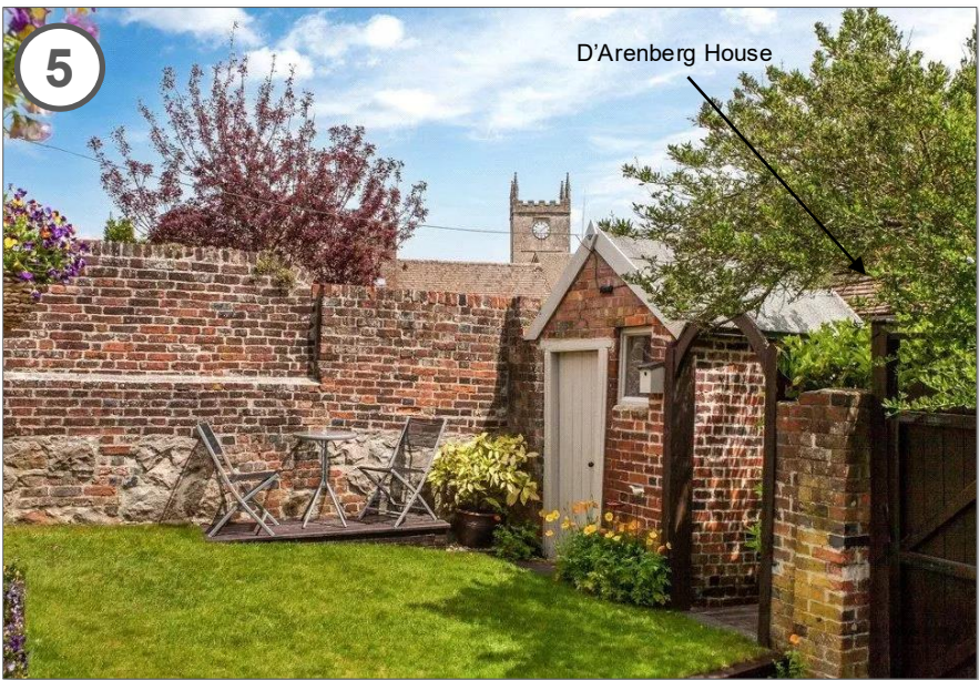
5. North-eastern boundary wall between The Nest & D'Arenberg House
