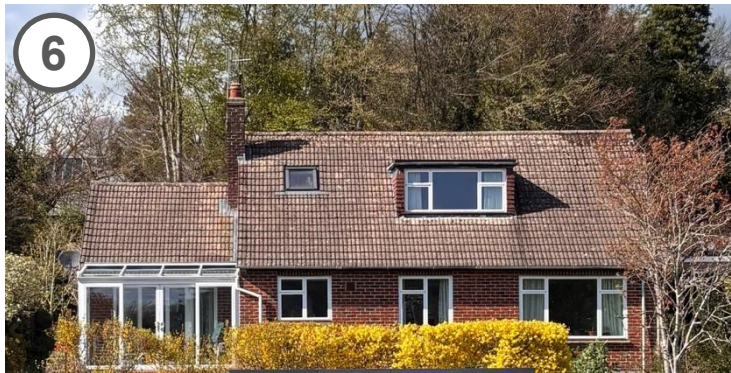
St Crispins box dormer facing north-west side of The Nest
