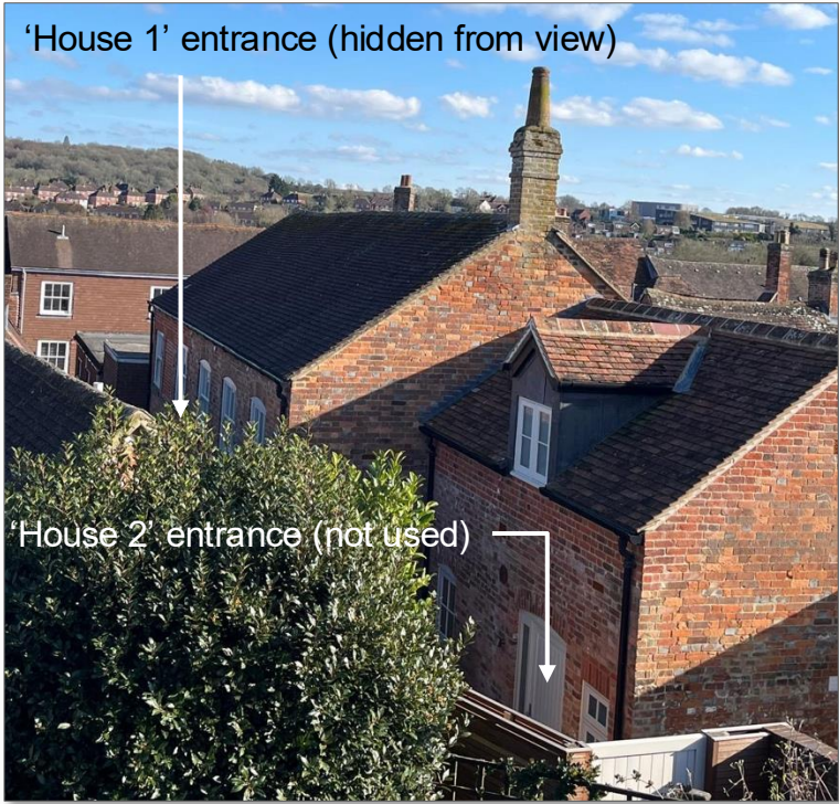
Four Candles roof as seen from roof of The Nest looking south
