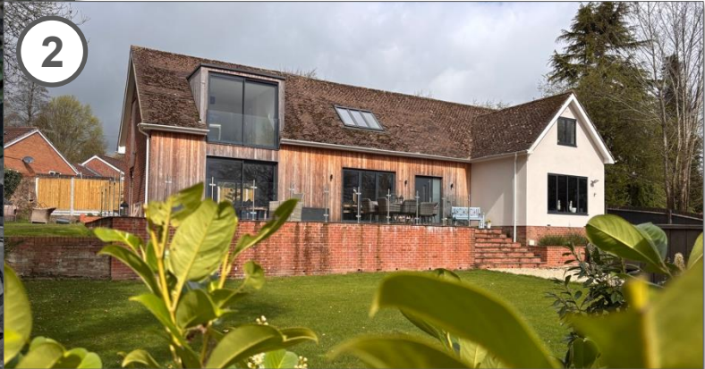
2. Sycamores (PL/2023/01654), Conservation Area, before & after recent modernisation
