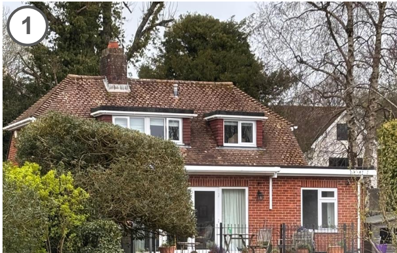
1. Linden House box dormers oblique to north-west of The Nest
