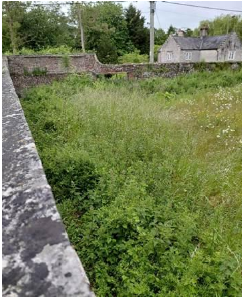
1. Photo of north side of entrance showing height of land and relationship to the Cotes listed western wall.
