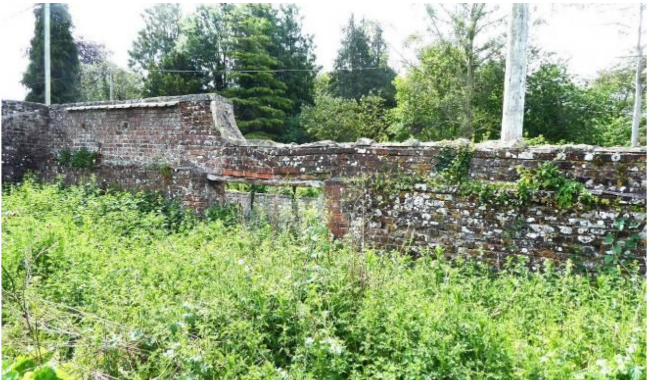
Gateway relative to 207 Boreham Road (left) – from field (north)
