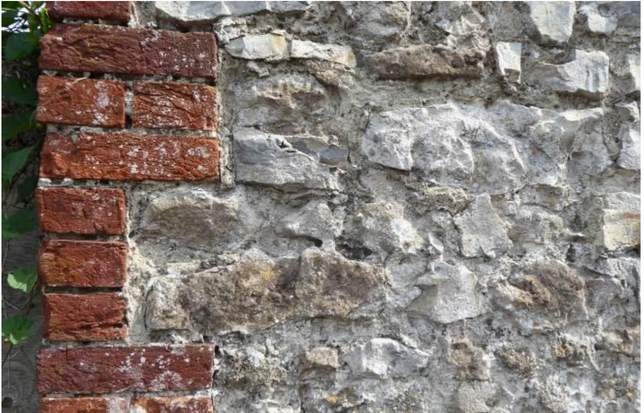
Wall face – road side (east jamb)
