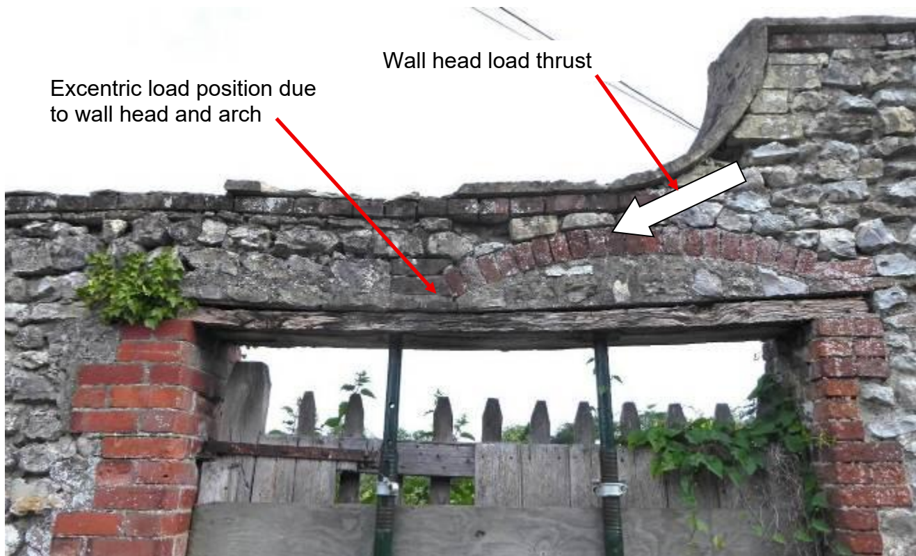
Gateway head – from road (south)
