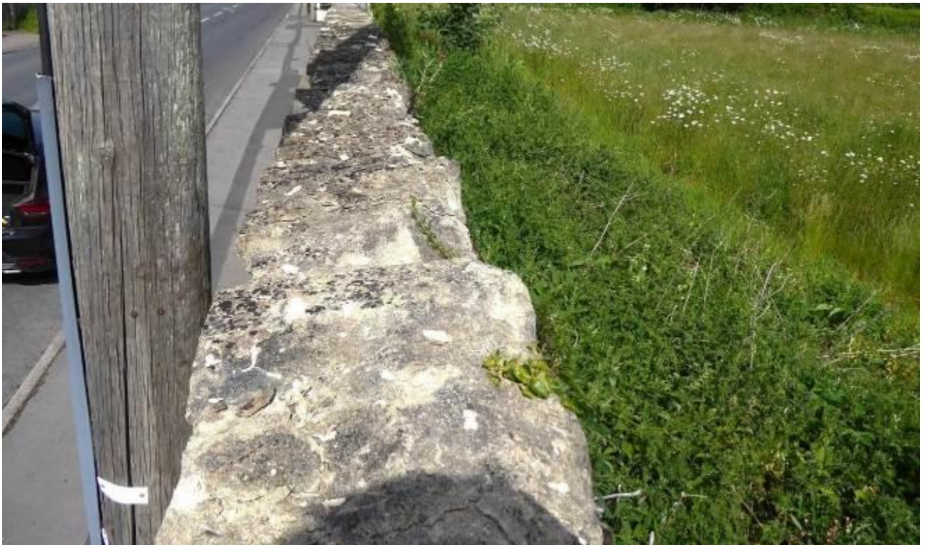
Coping condition – looking west
