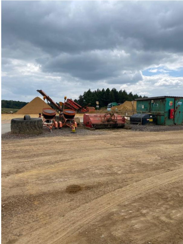
Figure 10: Quarry area showing stockpiled aggregate, equipment storage and compacted ground.
