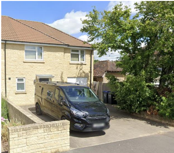
Front Elevation (Google Streetview July 2024)
