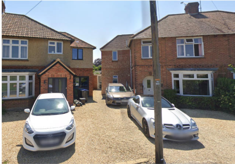
Two storey side extensions at numbers 16 & 18 Eastleigh Close
