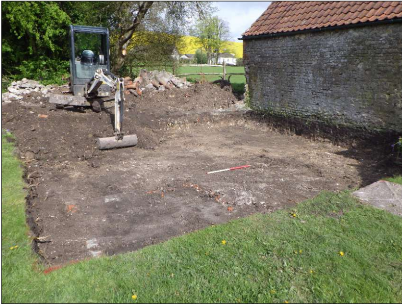
Plate 1: General view of site area during reduction, looking north (1m scale)
