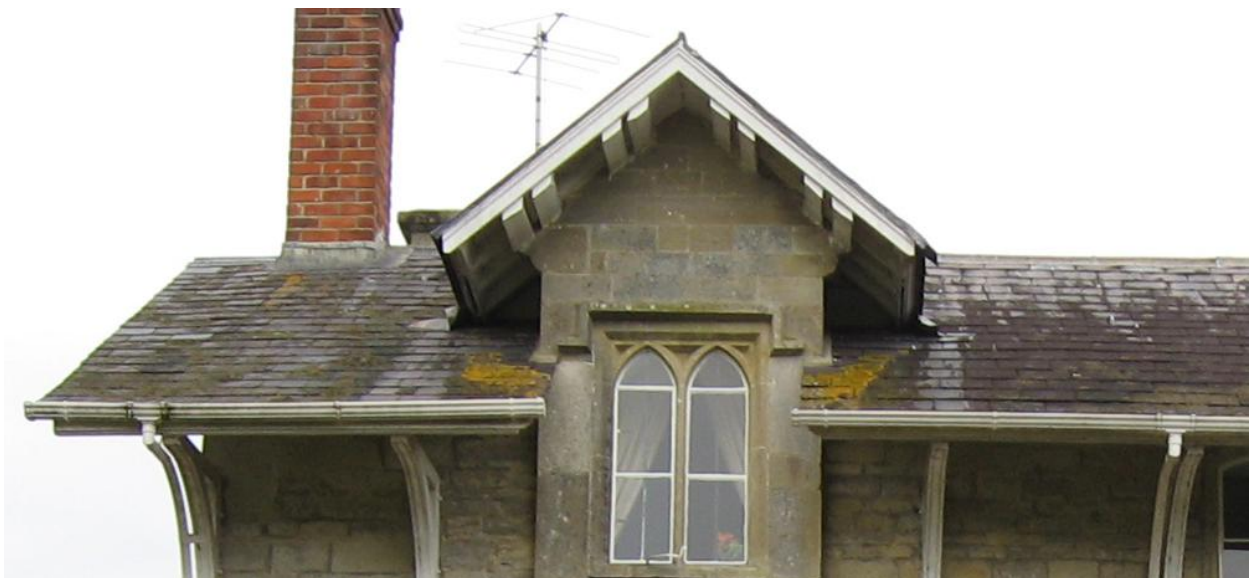
Roof of south range 2023
