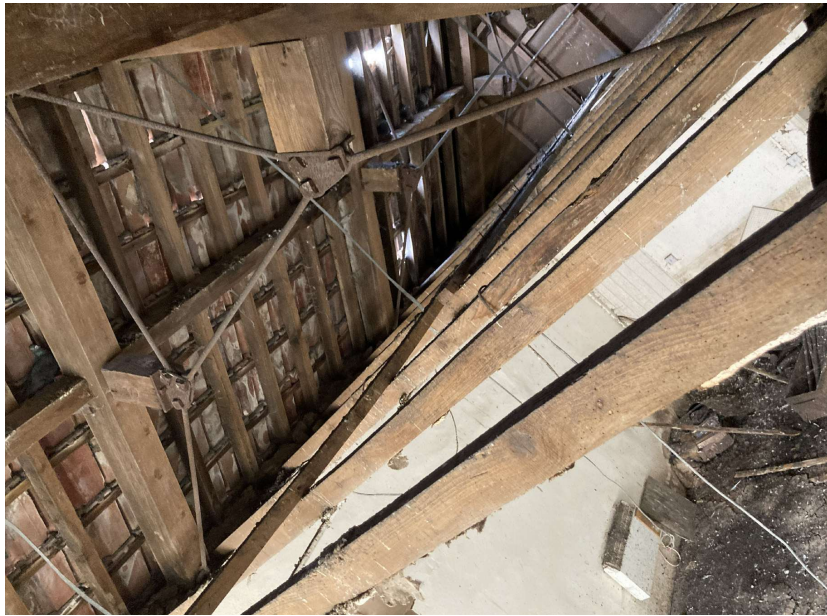
Existing roof trusses with metal tie rods and purlins between. Rafters over. Timber battens with double Roman tiles hooked over. Ceiling joists below, no ceiling currently. All roof timbers to be retained, splice repair made if required. Structural engineer to inspect the roof
