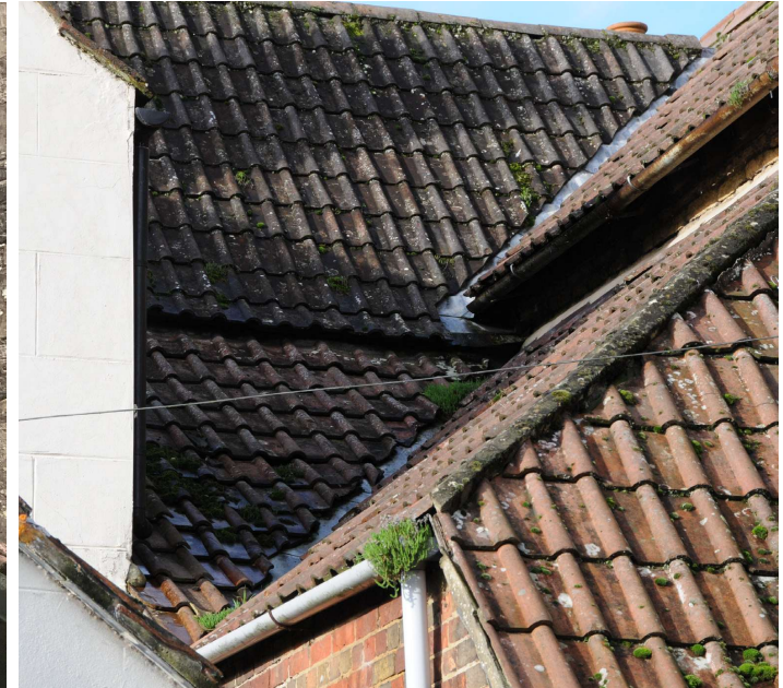
Existing lead valleys to be removed, the timber lay boards inspected and replaced before new lead installed
