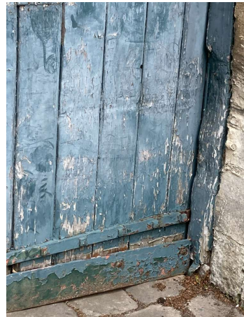
Existing ambulance station doors to be sanded back, repaired if necessary, primed and repainted to match the existing. New hardware
