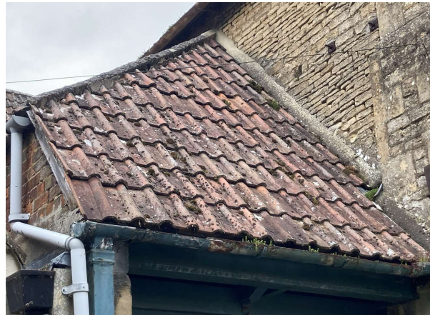
Existing front sloping roof to the ambulance station. Existing double Roman pantiles to be set aside for reuse. Mortar hip fillet and mortar fillet to wall abutment to be replaced with new lime mortar. Existing timber to verge to be replaced with new timber to match the existing.
