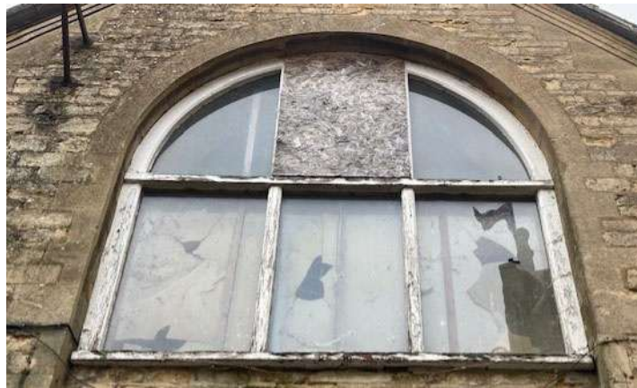
Existing large arched window to the first floor of the east elevation. Timber to be sanded back. New hardwood timber sill required. The rest of the timber to the window to be repaired with resin as necessary. All to be primed and painted to match the existing.
