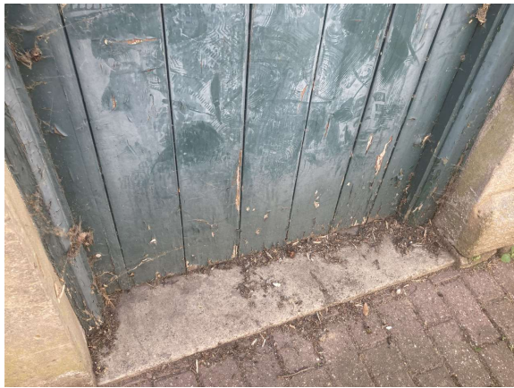
Existing door on to Patford Street to be sanded back, repaired if necessary, primed and repainted. New hardware
