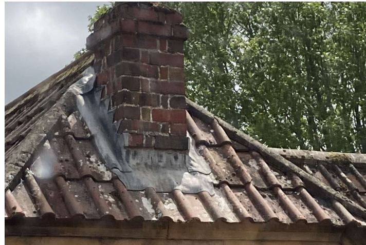
Existing brick chimney, leadwork to be renewed
