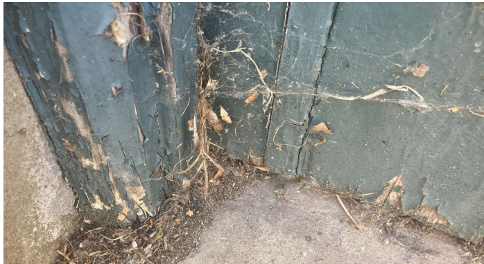
Existing door on to Patford Street to be sanded back, repaired if necessary, primed and repainted. New hardware
