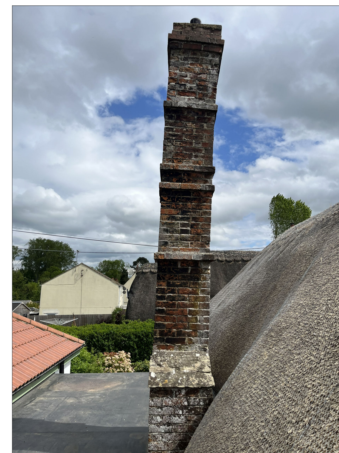
PHOTO OF THE CHIMNEY FROM THE WEST
