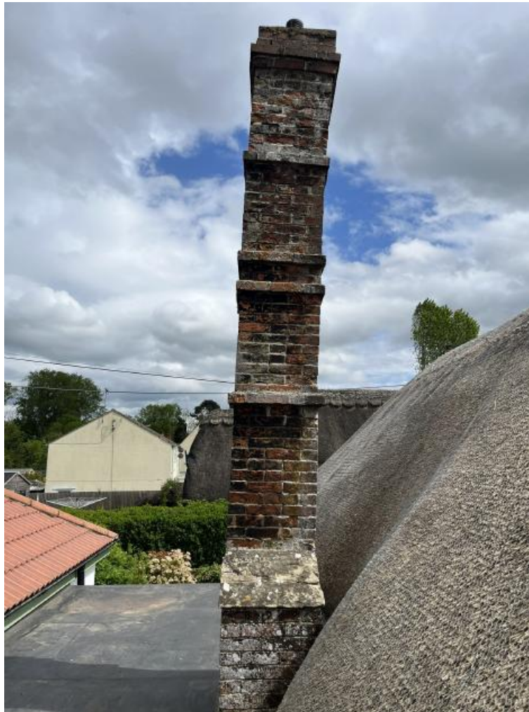
Figure 3 – Photograph of the chimney
