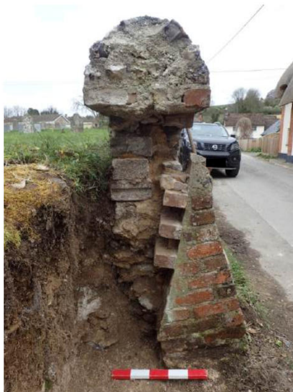
Figure 3. Cross-section of wall (1m scale, looking W)
