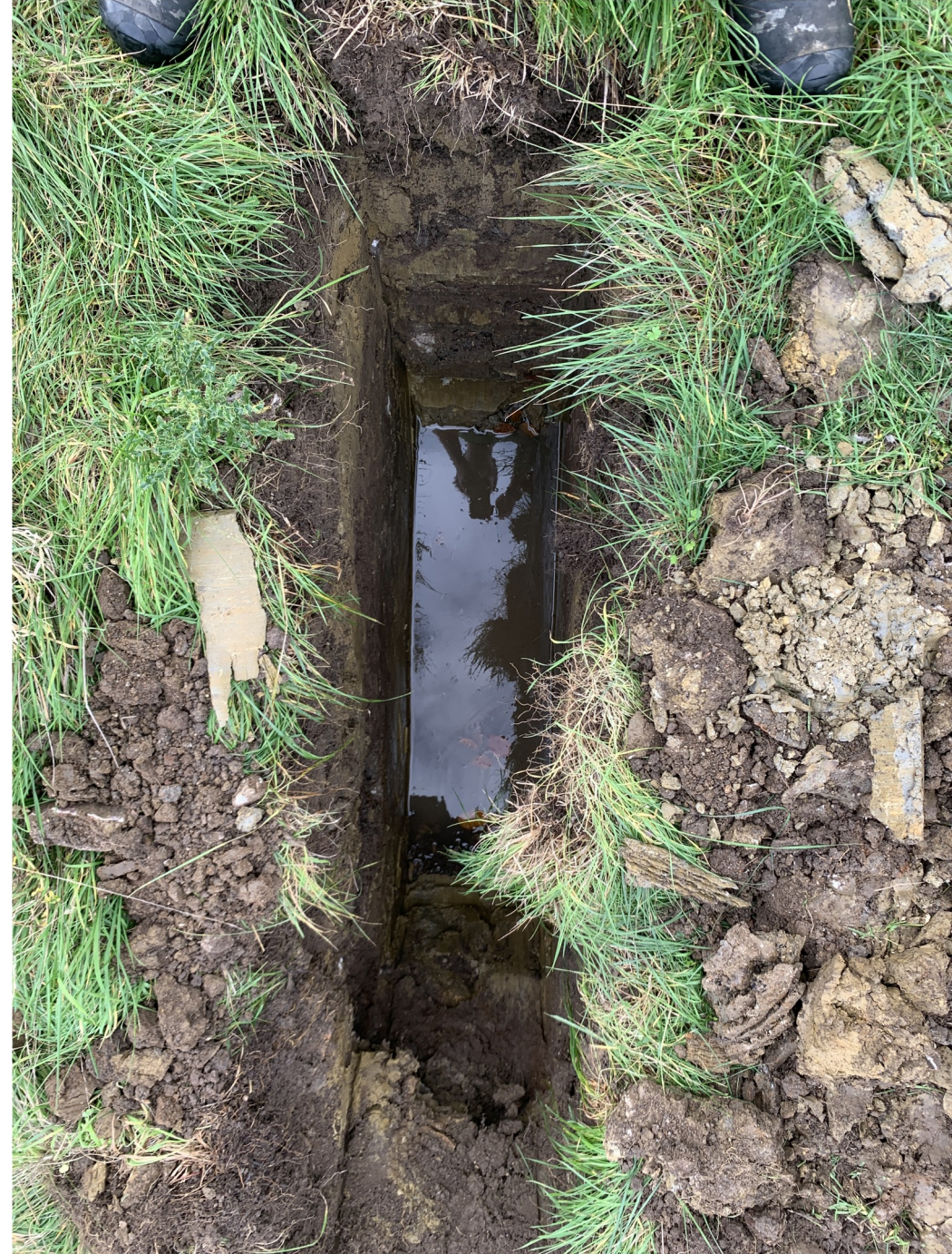
Area 2 - Soakaway Test Trial Hole
