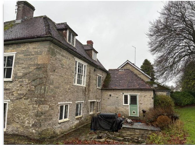
Figure 28. North elevation of main house, and east elevation of utility, with door and window opening.
