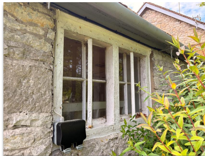
Figure 30. Easternmost window in north elevation of utility.
