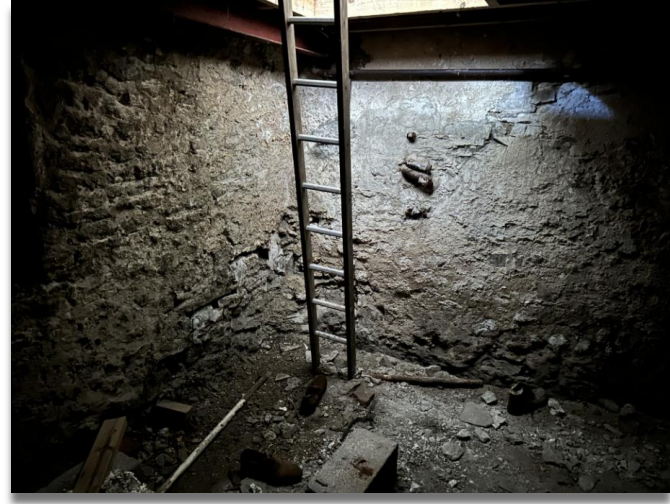
Figure 26. Cellar, note C20 steels and historic stair line.
