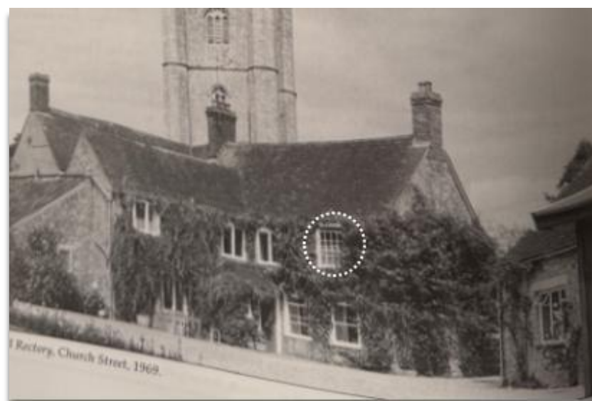
Figure 17. 1969 photograph capturing west elevation with first floor sash window.
