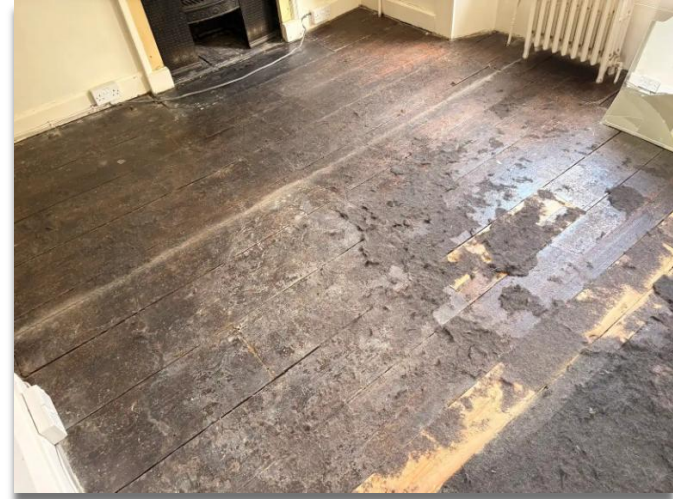
Figure 50. Bedroom 2. Ad hoc timber replacement.
