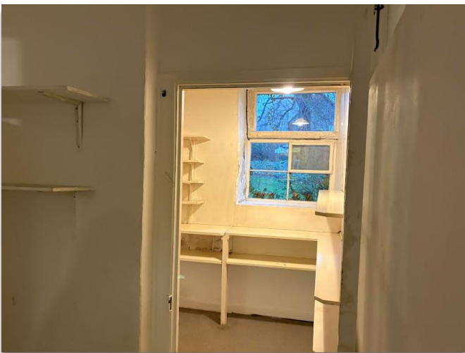
Figure 23. Existing utility looking north.
