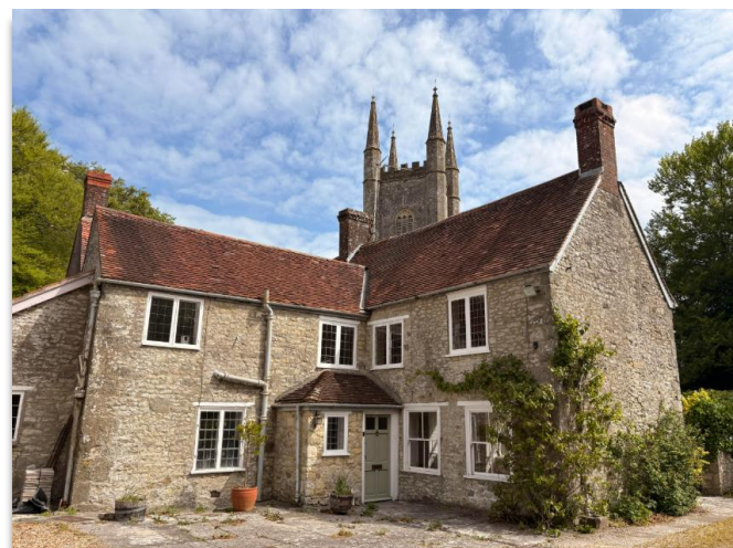
Figure 64. South elevation; note soil pipe and porch.
