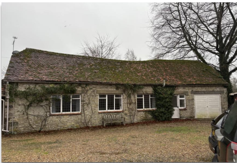
Figure 16. North west elevation of Field Cottage, former coach house/surgery.
