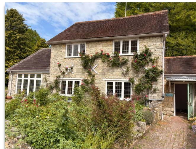
Figure 44. South elevation of Old Rectory Cottage and entrance lobby.
