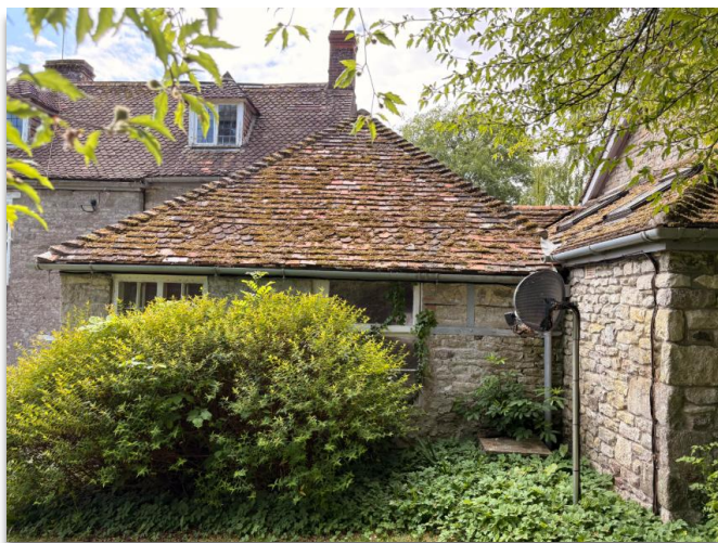
Figure 29. North elevation of existing utility.
