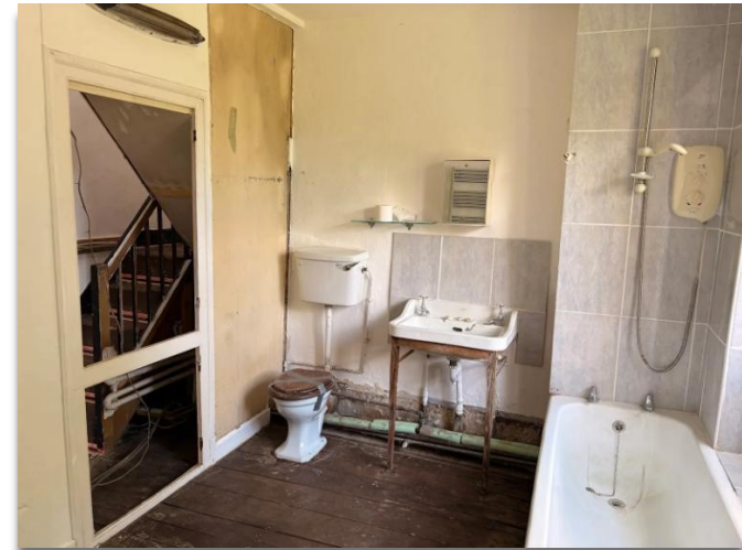
Figure 52. Bedroom 1 ensuite. Note lightweight partition.
