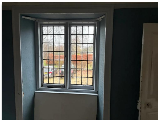
Figure 60. Bedroom 3, C20 replacement window.
