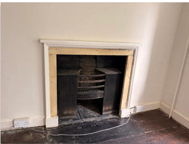
Figure 59. Bedroom 2; Georgian, cast-iron grate within fireplace.
