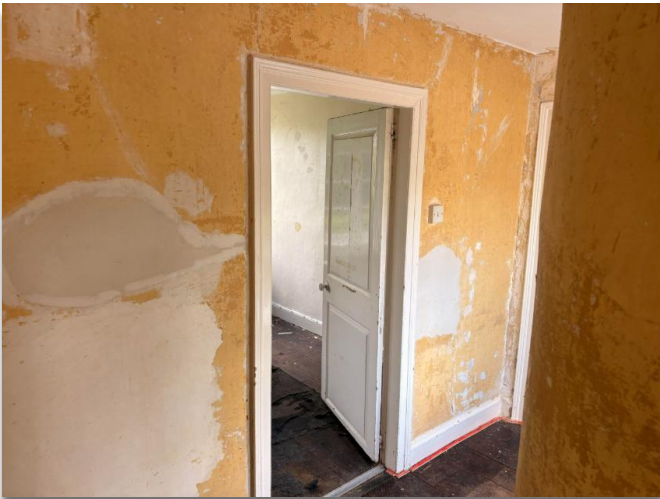
Figure 55. Bedroom 2 door from hall.
