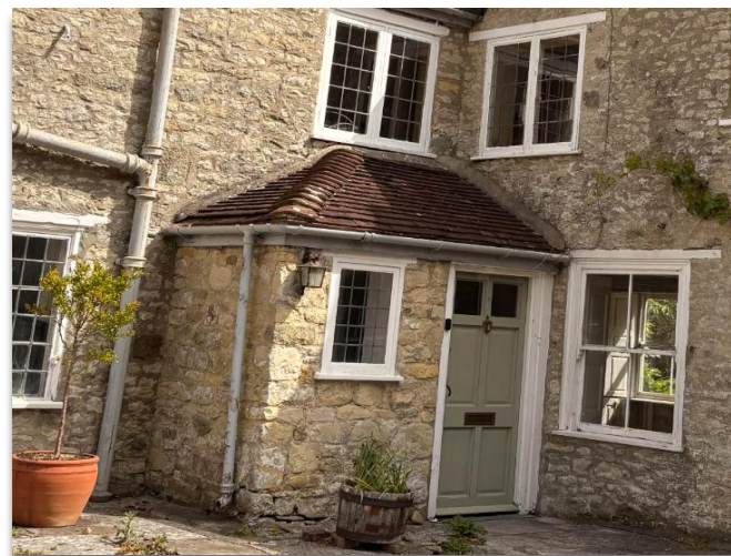
Figure 34. South and west elevations with porch. Note soil pipe.
