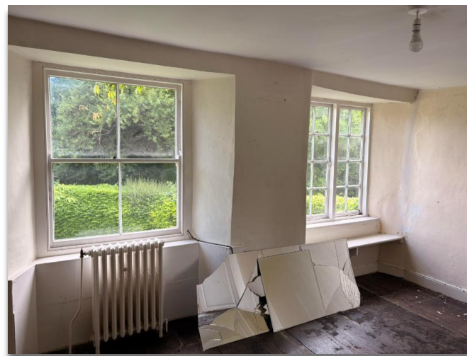
Figure 58. Bedroom 2 sash and casement windows.
