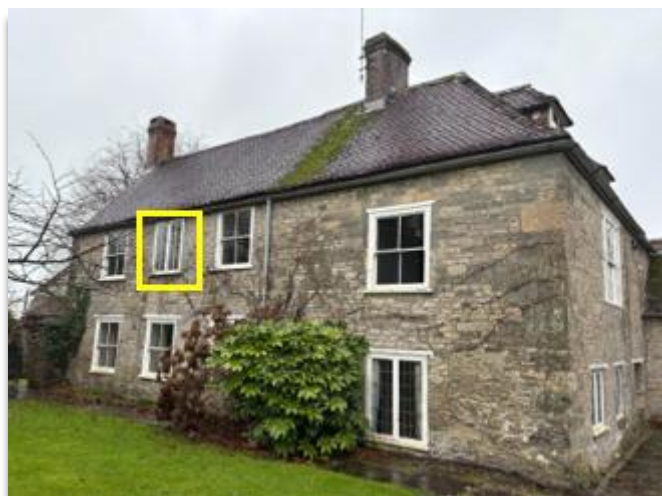
Figure 63. Central casement with glazing bars. Bedroom 2.
