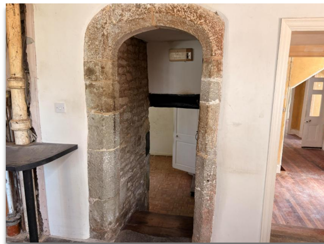
Figure 42. Looking towards snug and entrance hall from existing kitchen, through historic stone arch.
