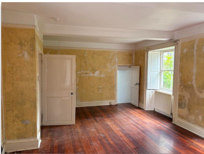
Figure 37. Looking north in drawing room. Note lobby to west (left).
