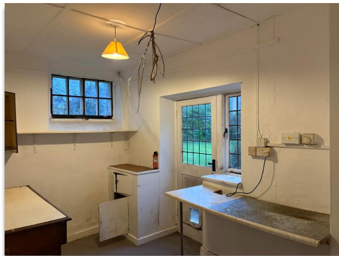
Figure 24. Existing utility, east and north walls.
