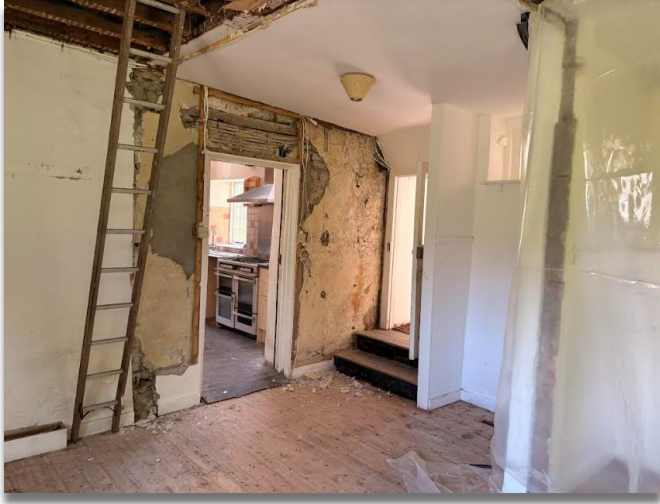
Fig.25. Existing utility looking south west. Note lintel above door.
