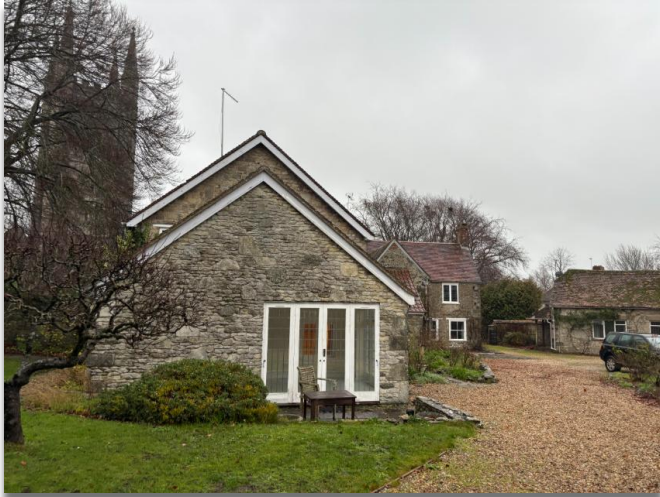
Figure 45. West elevation of Old Rectory Cottage (garden room).
