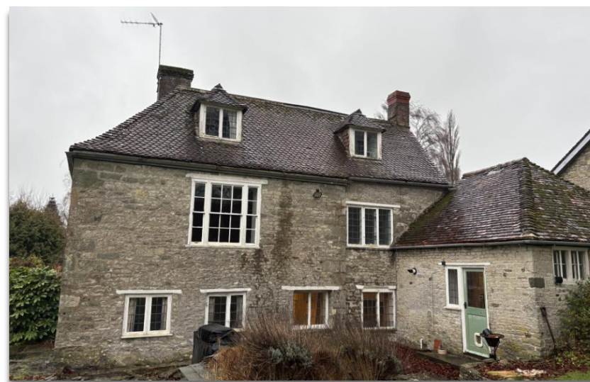
Figure 15. North elevation; earlier core within this range.
