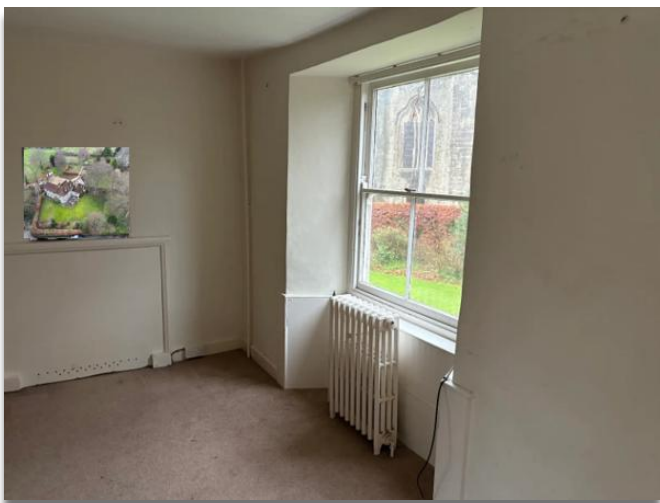
Figure 57. Bedroom 2; looking north east (note sash window and blocked fireplace).
