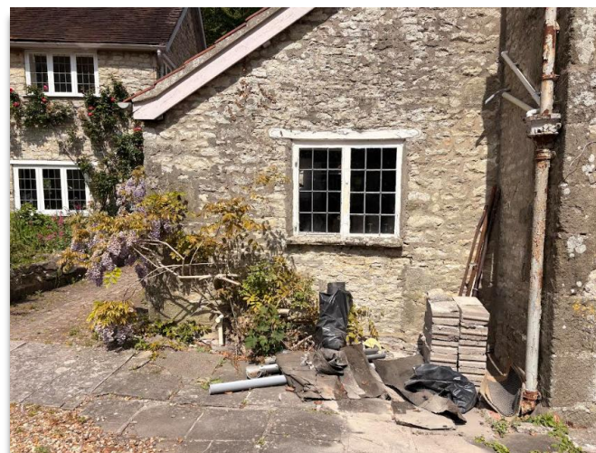
Figure 32. South elevation of existing kitchen, note evidence of blocked door (beneath window).
