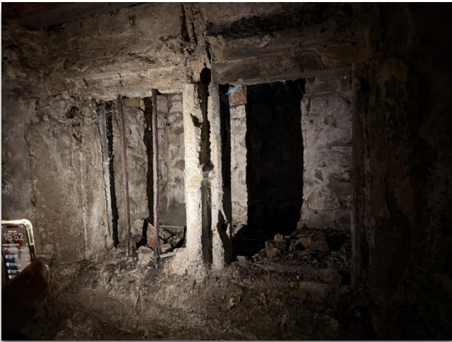
Figure 27. Cellar; opening with mullion and iron ferramenta.
