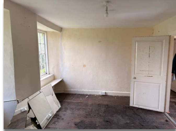
Figure 54. Bedroom 2; note door to hall and window.
