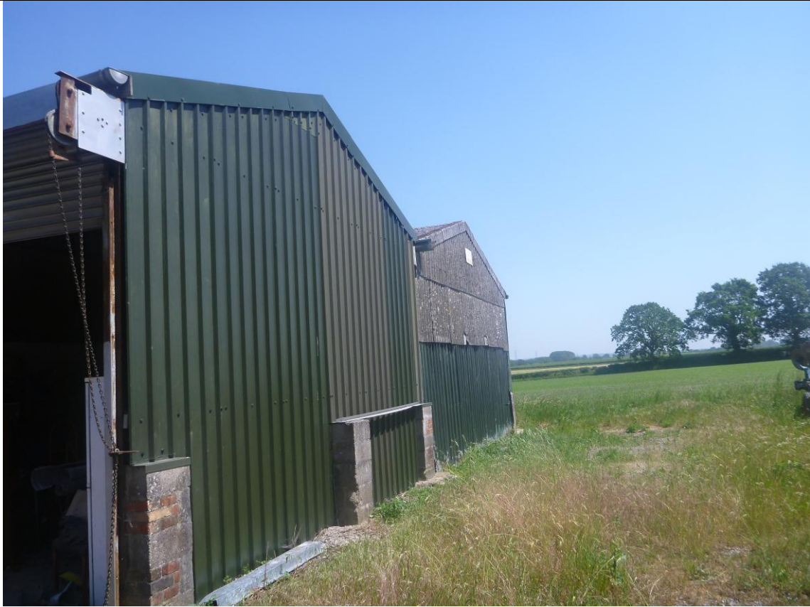
Fig 2: The existing barn is surrounded by bare ground with sparse vegetation, dominated by grasses.
