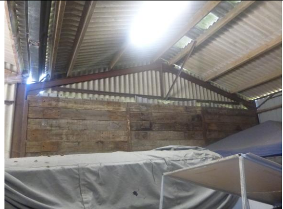
Fig. 4: The roof was untreated corrugated cement fibre sheets with no covering or roof void. One wall had untreated sleepers exposed while the rest were untreated corrugated cement fibre and untreated corrugated metal.
