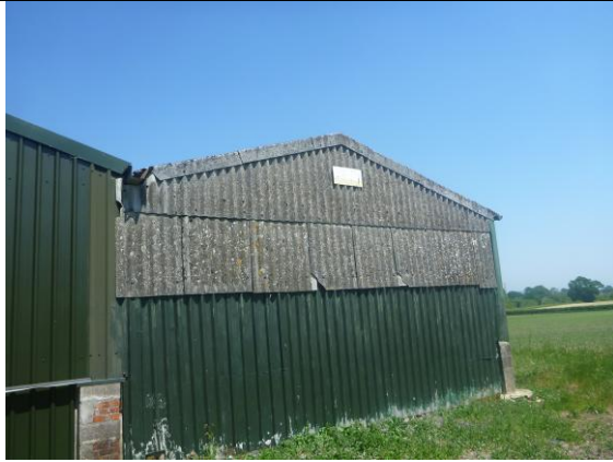
Fig 3: The existing barn is a double height steel frame with the walls made of untreated sleepers, blocks, untreated corrugated metal sheets and untreated corrugated cement fibre sheets.
