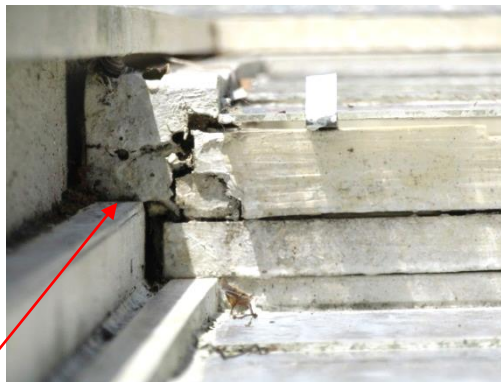
Sashes fail when the timber is rotted and there is no gap for the runner
