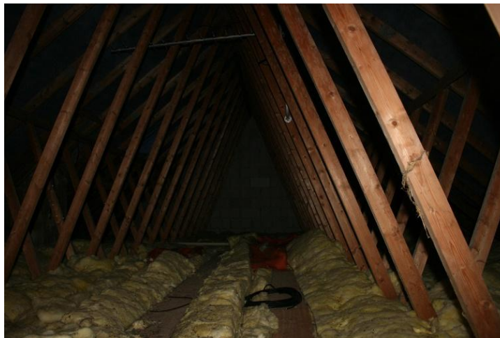
Photo 2: Inside the loft void.
