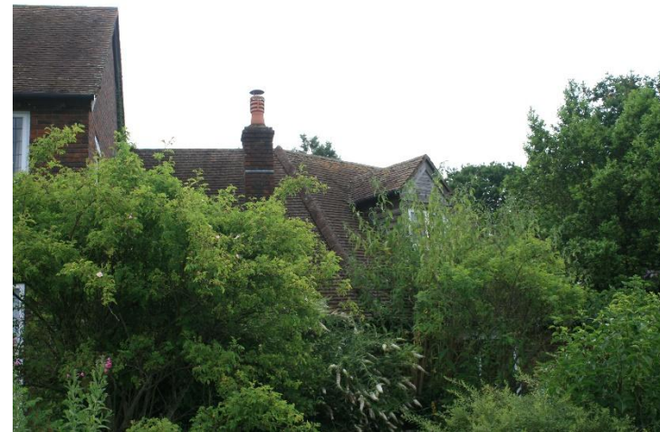
Photo 9: South elevation of the annexe (B1).
