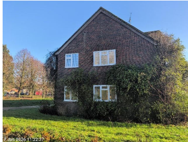
Photo 34: Western elevation of the house ('B1').
