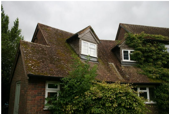
Photo 11: North elevation of the annexe (B1).
