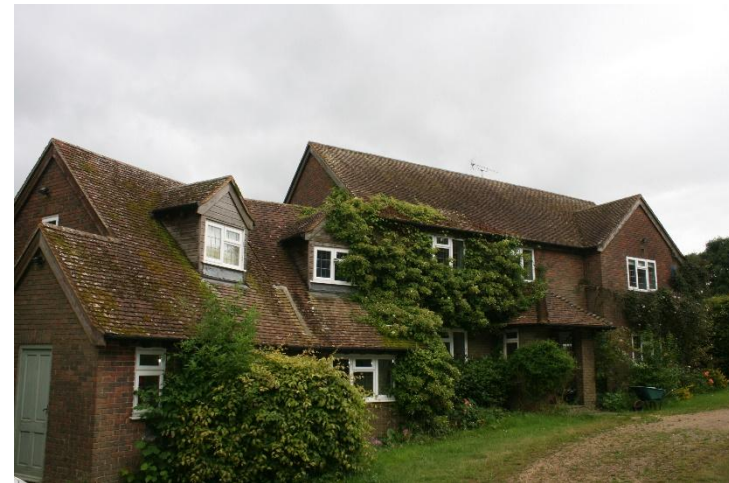
Photo 12: Northeast view of the house (B1).
