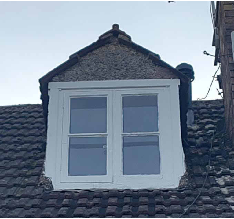
External view of existing rear dormer
