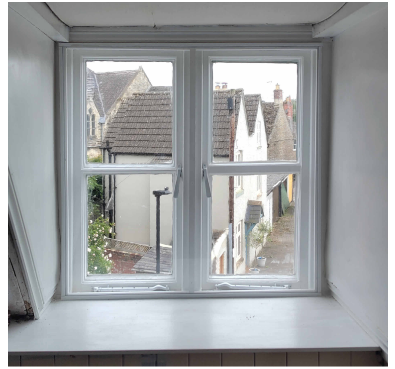
Internal view of west dormer.
