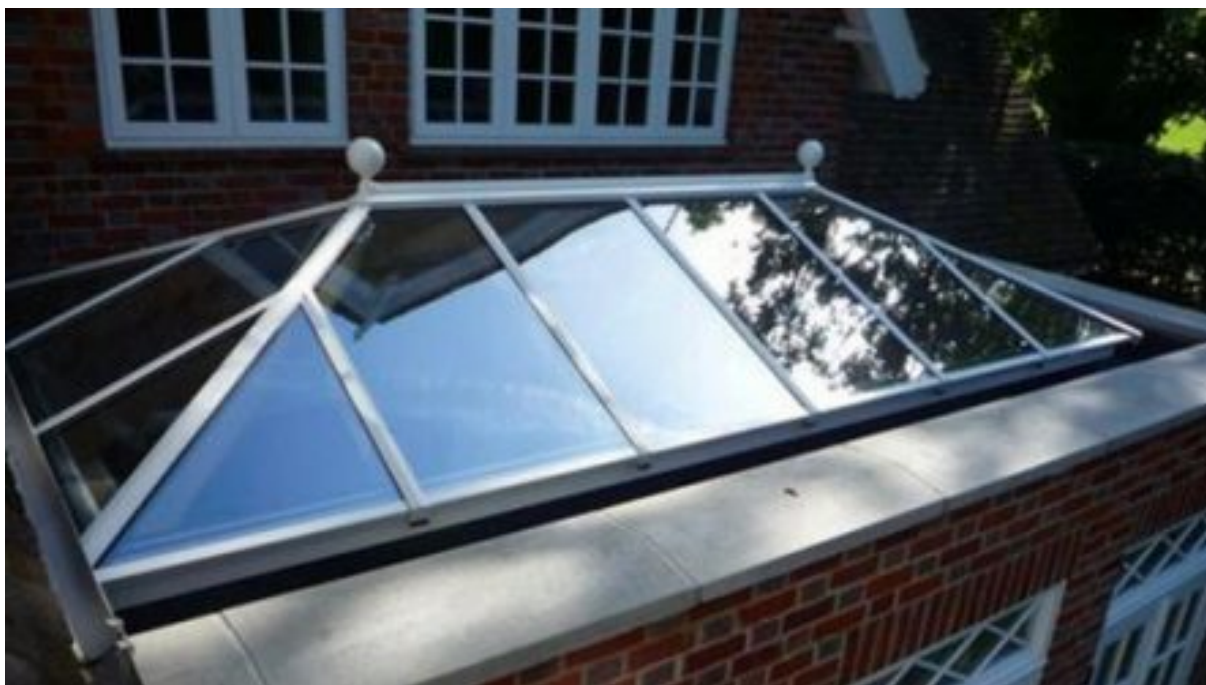
Roof lantern to flat roof
