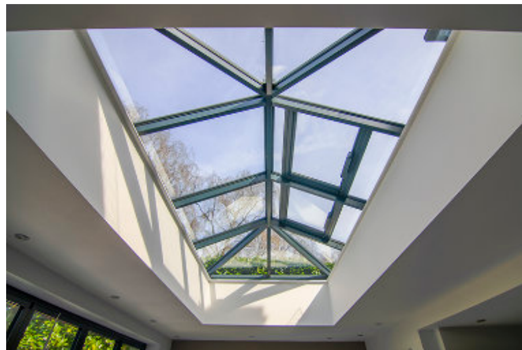
Roof lantern to flat roof
