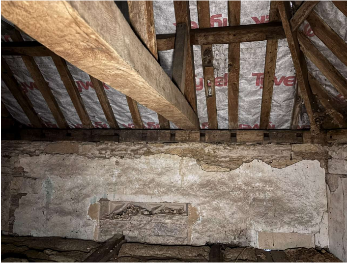
Internal face of eastern wall showing redundant pockets in wall plate – suggesting possible previous ceiling level.
