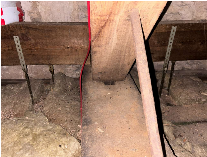
Tension rod through the strut
