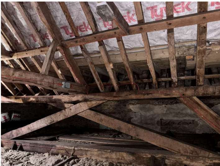
Girder truss beneath valley with roof structure over
