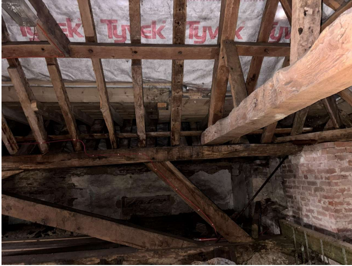
End of girder truss showing arrangement of struts and tension rod
